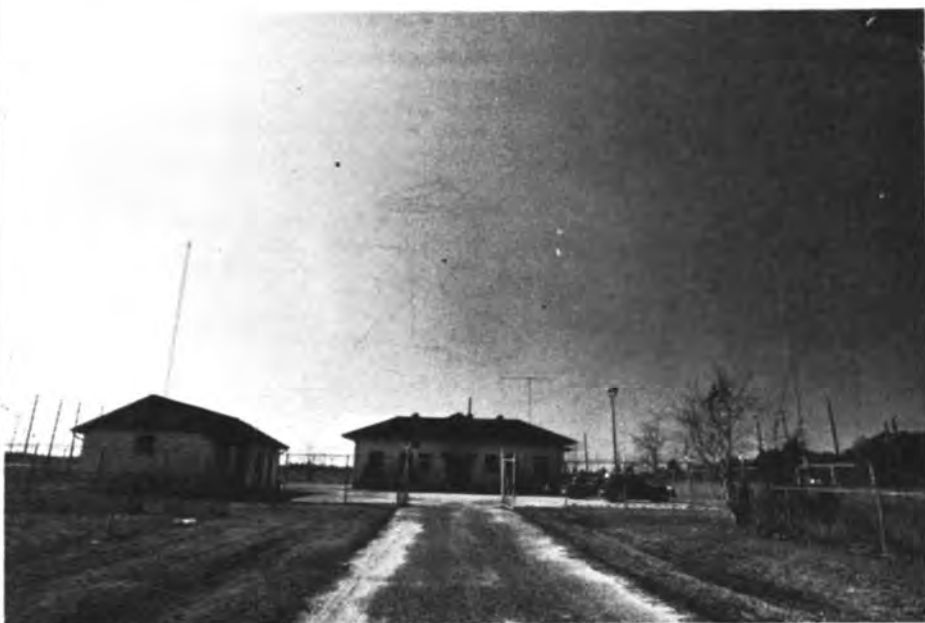
WNU External view of Slidell Radio Transmitter site, located off Ganse Road, Slidell, LA. In background WNU's 150 ft. towers which support medium frequency 400 foot long double wire "T" antenna. Elsewhere are portions of 'doublets' and rotatable beam.
